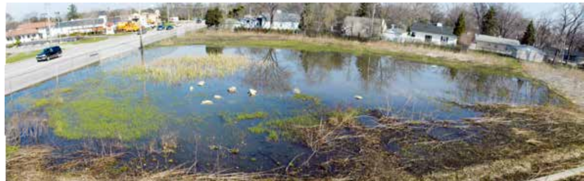
The Milwaukee Avenue swale at near maximum depth following a prescribed burn that removed almost all debris. Image acquired using a wide-angle lens from the roof of the Interpretation Center.
